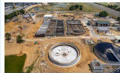
SANDHILL UPGRADE COMPLETED
