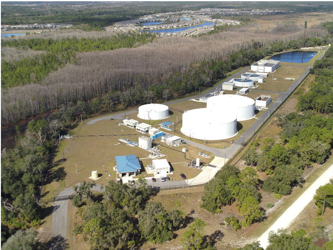
Sunbridge Wastewater Reclamation Facility
